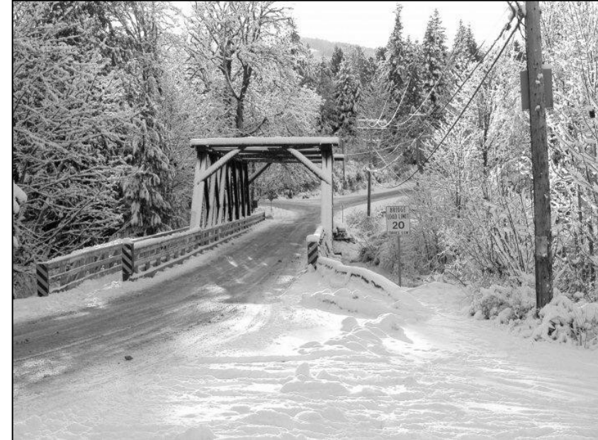
Cowichan Station Bridge – Dave Beddows
